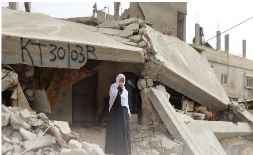
Figure 2.7 An assessment for such a house is (full destroyed). (OCHA, 2014)
